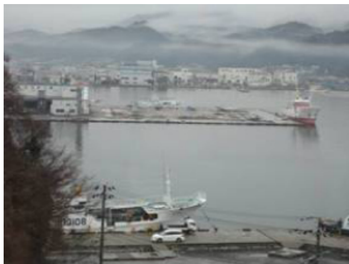
Fig. 1 Subsidence of lands, Kesenuma
