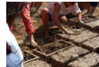
Fig. (1.1): Mud clay and straw are mixed and pressed into moulds
