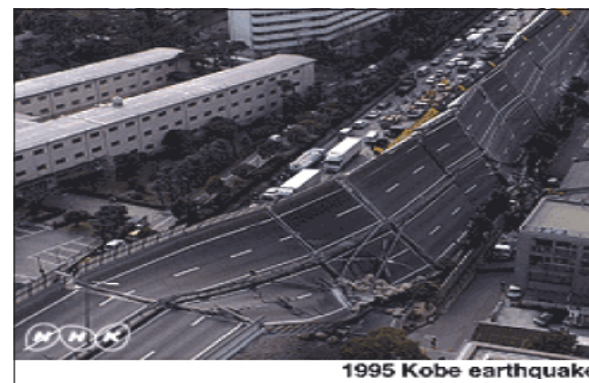
Fig.4 Kobe EQ:95- Extensive Damage to Transportation network. (Total Loss- $150 B)
