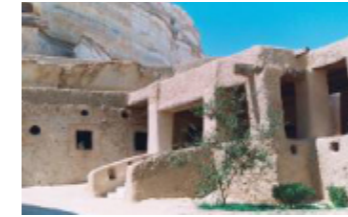
Fig (8.1): The entrance with small windows to capture the prevailing wind
