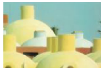
Fig. (4.2): Sheraton Miramar Main hotel by Michael Graves
