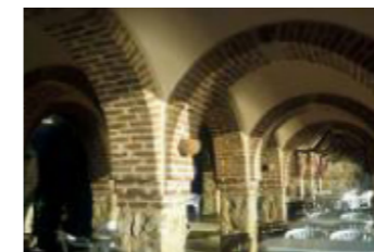
Fig (3.1): Masonry view, seating area (Quseir Movenpick), Egypt
