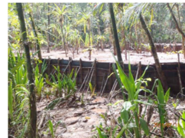
Fig.5 The easy fence for protecting clay runoff
