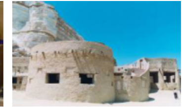
Fig (8.6): The rough texture of the building plaster creates shaded areas on the facades
