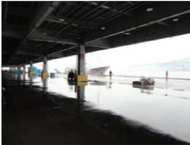
Fig. 7 Buildings remained at Kesennuma
