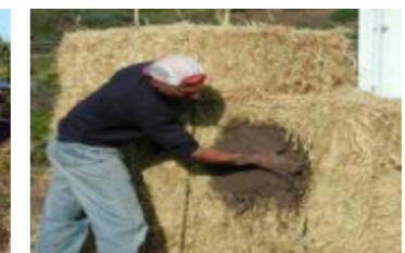
Fig (2.3): Building with straw bale
