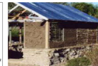
Fig (2.2): Exterior walls are built with straw bale
